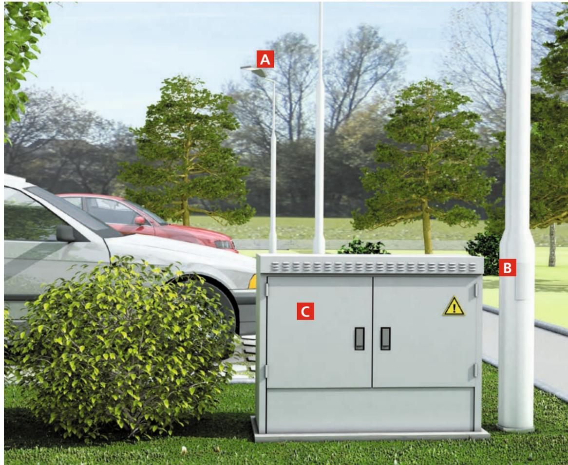
Indirect lightning discharge produces surges which far exceed the surge immunity of LED luminaires. This can lead to partial or complete failure of the LED module and defective LED drivers. Surges in the grid may result in the premature ageing of LED modules.
