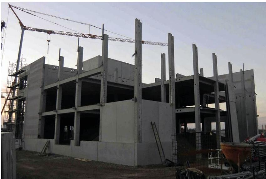
Figure 1 Reinforced steel supports as natural down conductors
